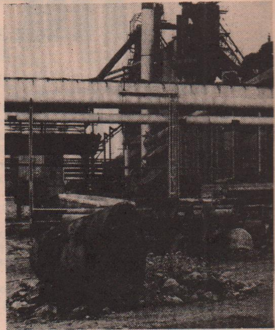
Steelworks under demolition in Scotland
